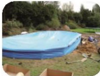
**Step 6** Hang the liner in position and begin to fill the pool.
