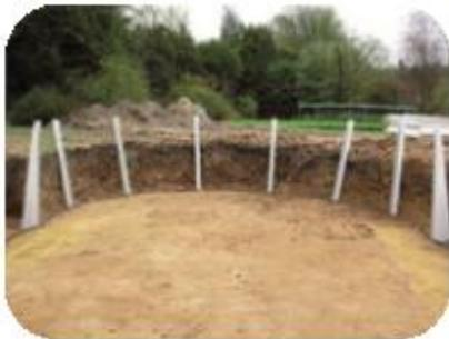
**Step 3** Lay the bottom rails round the pool the add the verticals.
