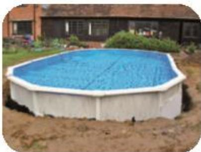
**Step 7** Once the pool is full of water, connect the filtration.
