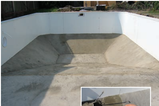
Day 8 - Screed The Base
