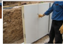
Day 4 - Installing the insulated panels
