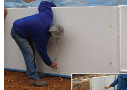
Day 4 - Installing the insulated panels
