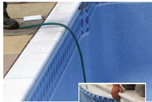
Day 16 - Install The Liner
