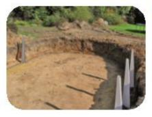
**Step 2** Put the com- pac support systems in the ground, then level the ground removing all sharp objects.
