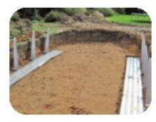
**Step 1** Firstly dig out for your pool allowing room to work around it, begin to build the Com-pac support system.
