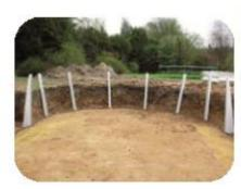
**Step 3** Lay the bottom rails round the pool the add the verticals.
