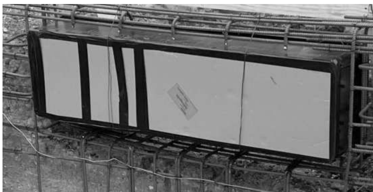
Image 4 BADUJET Turbo - Jet placement in rebar
